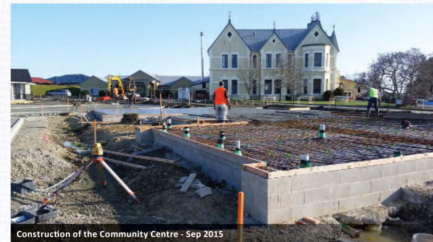
Construction of the Community Centre - Sep 2015
