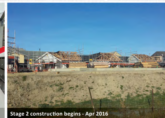
Stage 2 construction begins - Apr 2016
